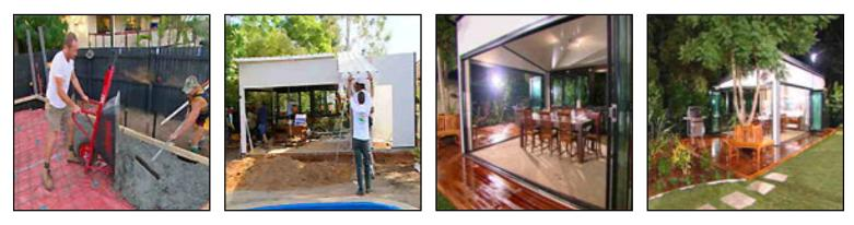
**Electrical trench:** Nigel and Jody dug a trench 600mm deep for power to the pool and we also utilised this trench for our new water line. We separated the water pipe from the electricity with 300mm of backfill. Always use a licensed electrical contractor.
